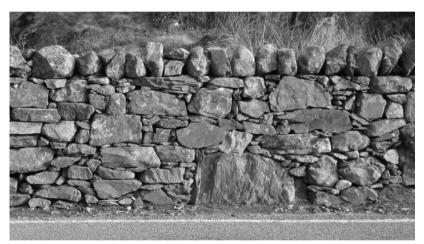
The wall left probably illustrates a complete lack planning and forethought (and probably a failure to basic grasp principles). Pins. plates, joints, poor grading and stone selection. Deciding where to begin with this sort of analysis is a bit of a problem. Essentially I will be trying to look at a small number faults and problems and how thev
