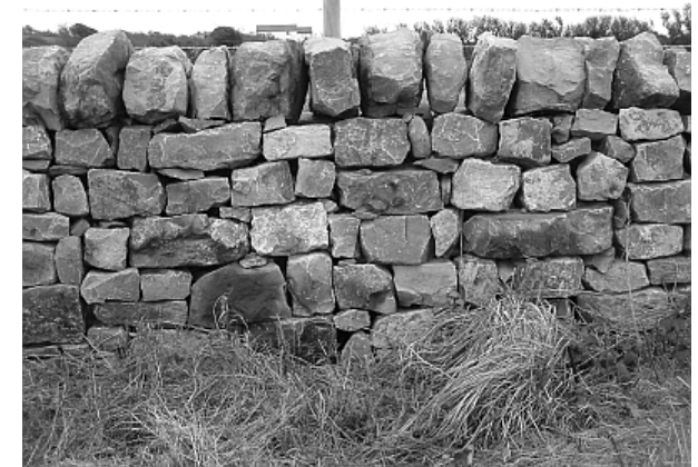
Complete running joint (centre). A5/A55 Anglesey
