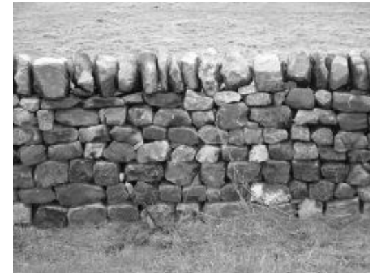
Complete running joint (centre). A5/A55 Anglesey
