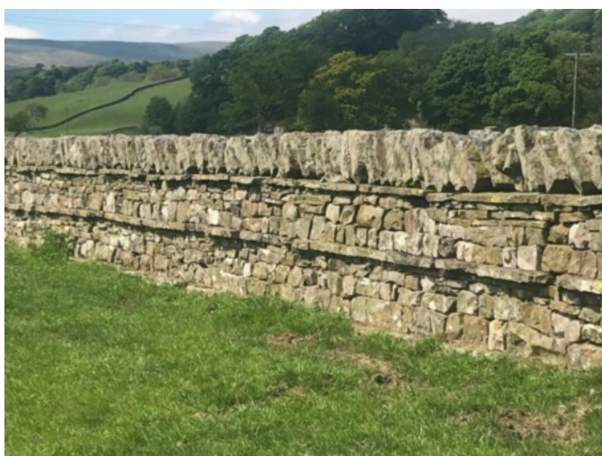
Complete layer of throughs (coverband under copes)
