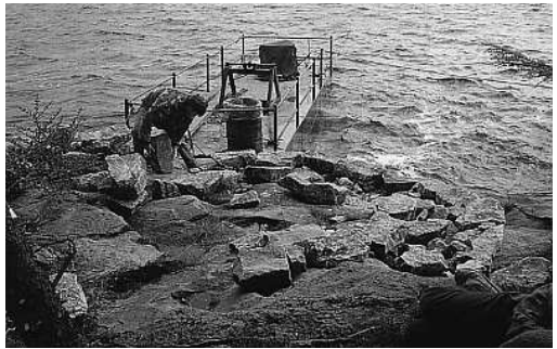
Temporary jetty and foundations © Chris Drury “Silent Spaces” Thames & Hudson 2004 . p116
