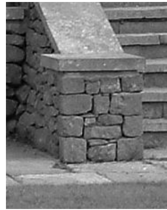
These three pillars on a site in Northamptonshire, are built of a brown limestone from near Banbury. The quoins are hand dressed and rarely more than twice as long as high often little more than cubes, hence by necessity the pillars have a mortar core.
