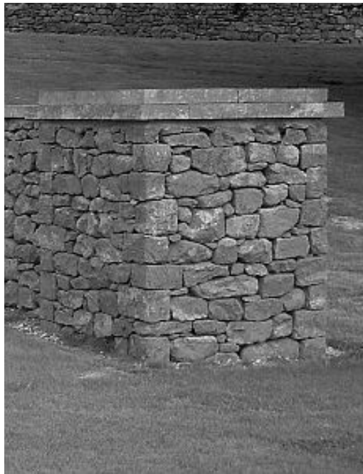
These three pillars on a site in Northamptonshire, are built of a brown limestone from near Banbury. The quoins are hand dressed and rarely more than twice as long as high often little more than cubes, hence by necessity the pillars have a mortar core.
